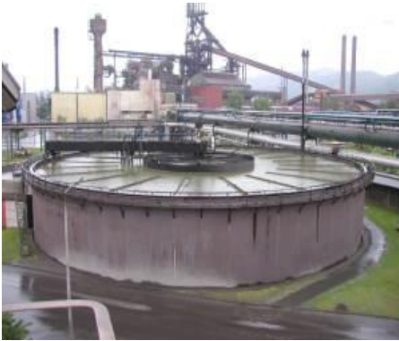
voestalpine Steel Division
